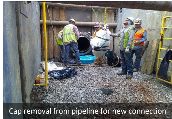
Excavation with trench boxes for safety
