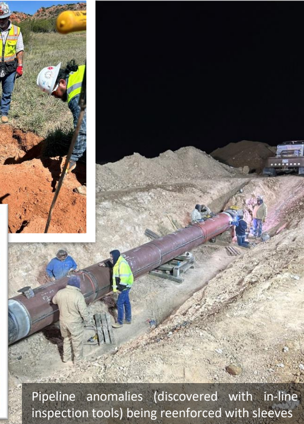
Excavation to evaluate anomalies and remediate pipeline damage as needed
